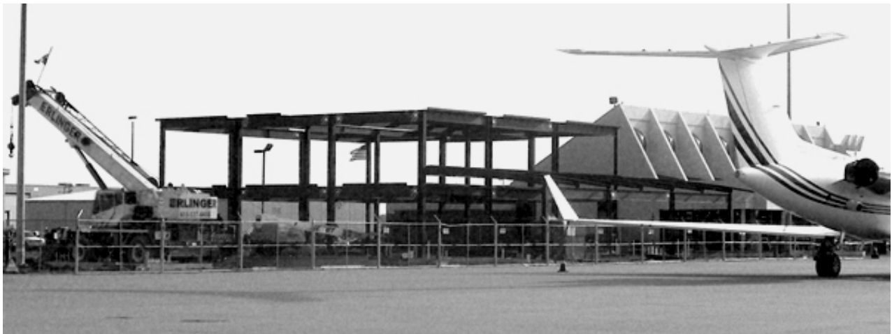
AIRPORT FIRE STATION CONSTRUCTION CONTINUES ON SCHEDULE
